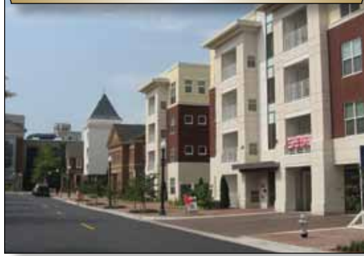
MONTICELLO STATION AT WELLS FARGO / Norfolk, VA Award of Merit
